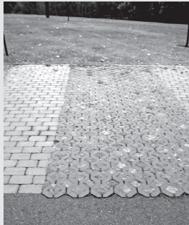
These grassy pavers are in Vajxo, Sweden, the "greenest city" in Europe. The pavers provide support for parking vehicles, while the grass growing within helps water drain and creates a natural appearance. The solid sections act as parking lines and give a solid surface to step onto.
